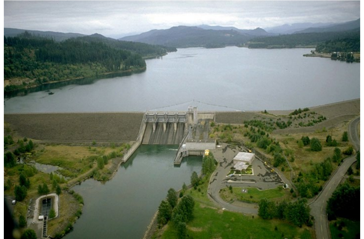
Foster Dam – USACE file photo
